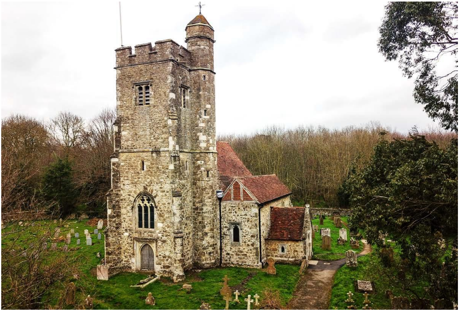
Photo: March 2018 – St. Martin's Church in Ryarsh located just a few hundred metres from the proposed site. Public footpaths link the surrounding villages and the new developments; Ryarsh Park and Leybourne Chase, to the church.
